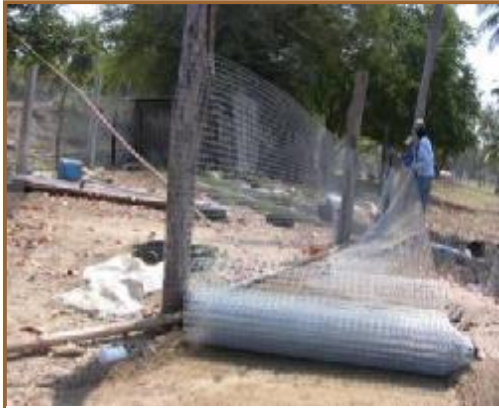
Building a new chicken house
